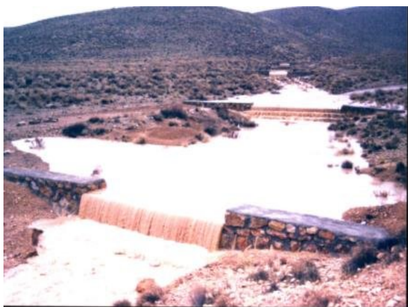
Fig3. Brick, Stone masonry checkdams
