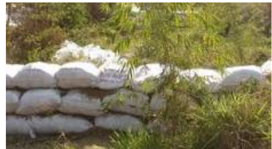
Fig2.Earthen and bori bunds/sand bag checkdams
