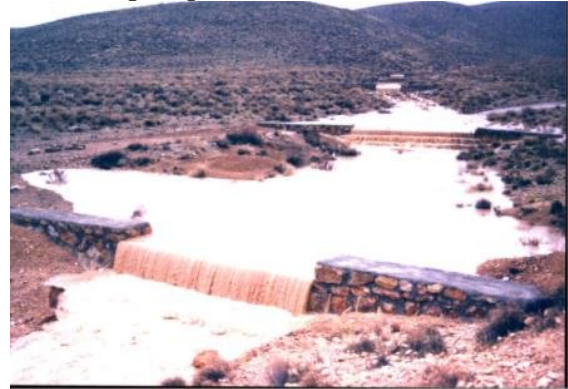
Fig3. Brick, Stone masonry checkdams
