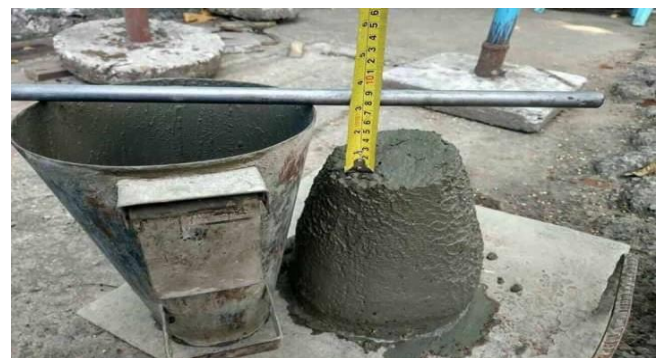
Fig. 1 Concrete slump testing
